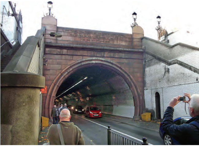
Rotherhithe Tunnel north portal
